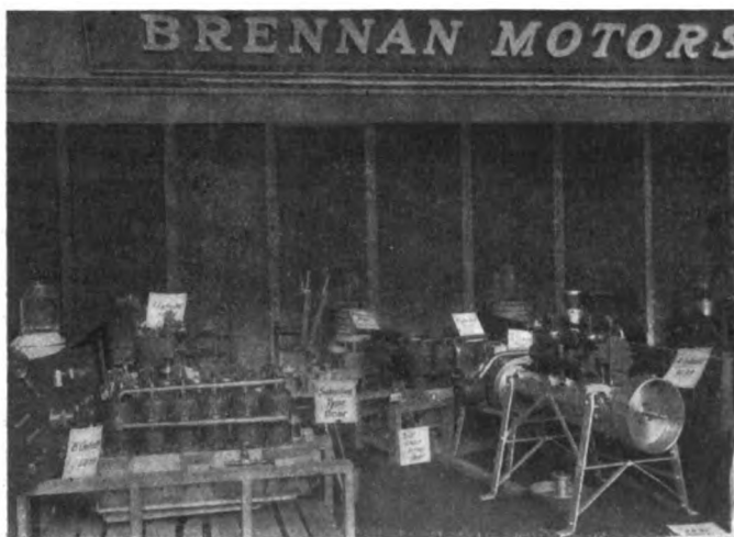
Engines and Transmissions from the Brennan Works.
